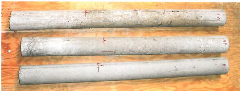
Photo 5c. Concrete From Pole Sections, Reassembled After Inspection.
