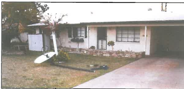
Photo 1a 2 . Broken pole in yard.
